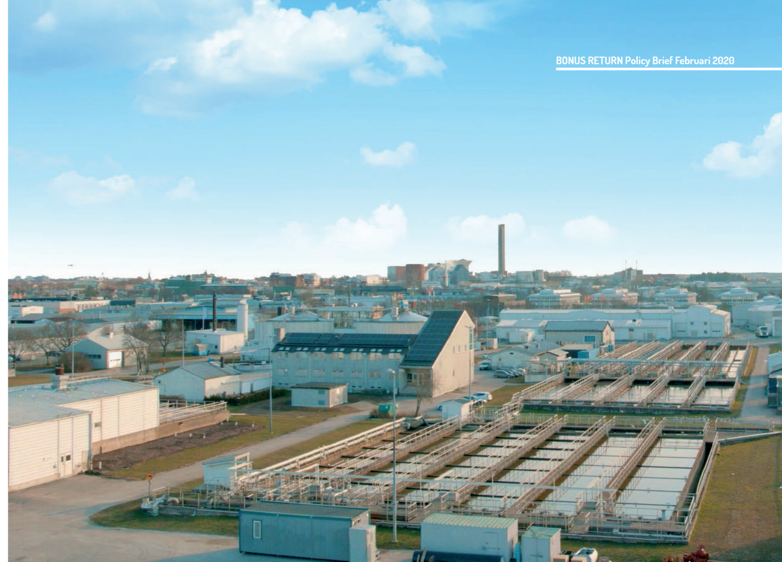
Uppsala wastewater treatment plant. Image: SEI
